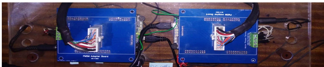
Fig 2.12: Connecting the The two inverter boards to the DC Supply
